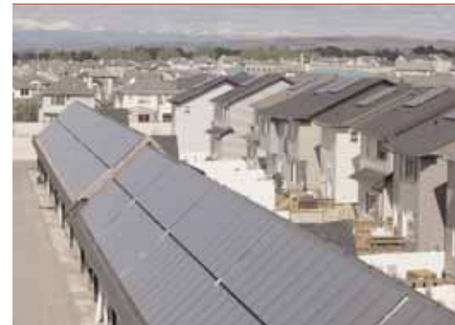
The Drake Landing Solar Community in Okotoks, Alberta
