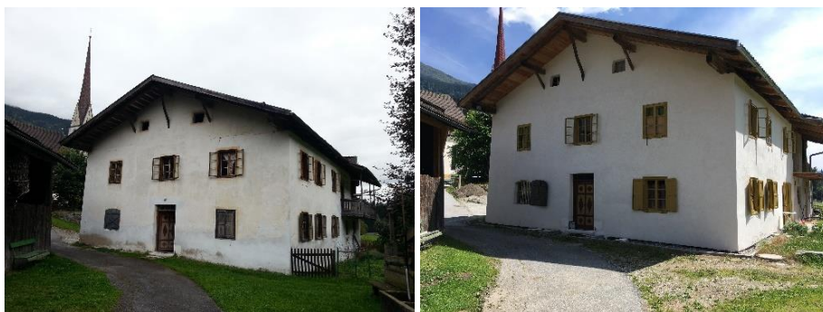
Figure 14: South view before and after retrofit, © Elmar Gruber
