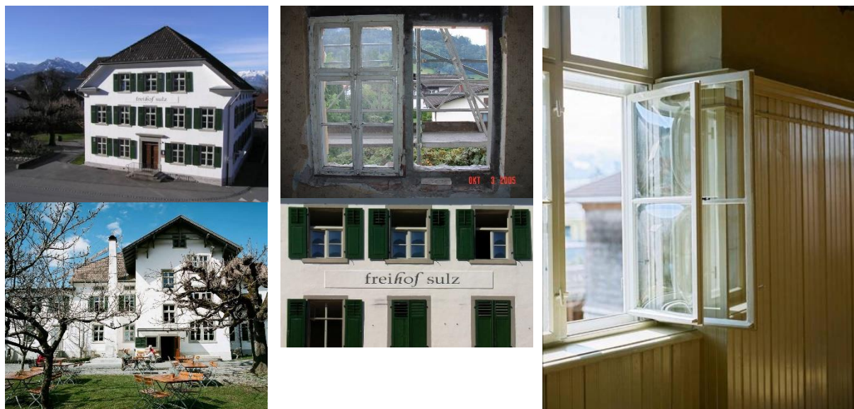
Figure 13: Window solution at Freihof Sulz before (middle above), © Martin Rhomberg, Beate Nadler-Kopf; and after renovation (box-type window), © Lukas Schaller
