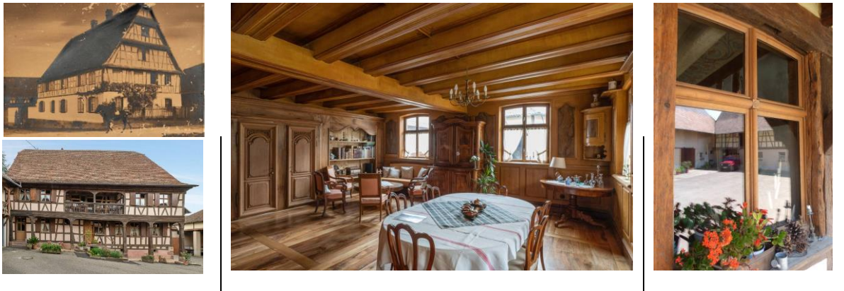
Figure 41: Timber-framed house in Alsace (single window) – before and after renovation.
