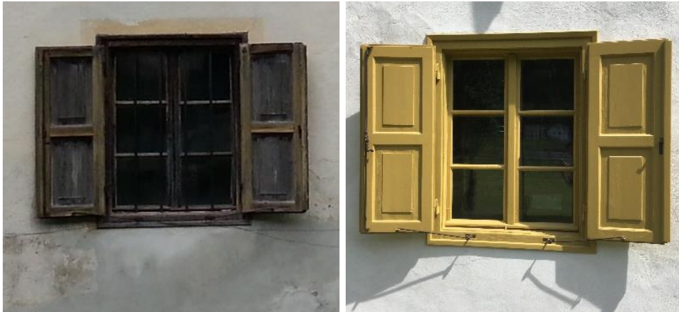
Figure 16: Knablhof (box-type window) – before and after renovation, © Darius Richter
