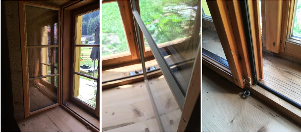
Figure 18: Knablhof (box-type window) – details after renovation, © Darius Richter
