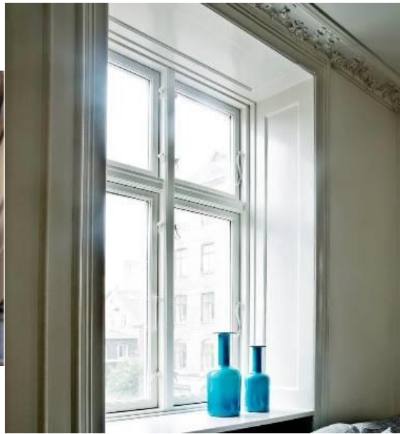
Figure 9: Left: Before renovation, the windows gave rise to condensation, draught and had a very negative effect on the indoor climate. Right: After the renovation, the new windows improved indoor climate significantly (Source: Leif Rönby).
