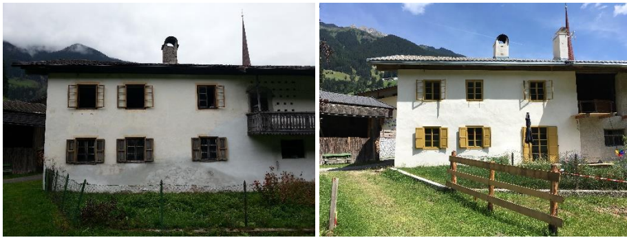
Figure 15: West view before and after retrofit, © Elmar Gruber
