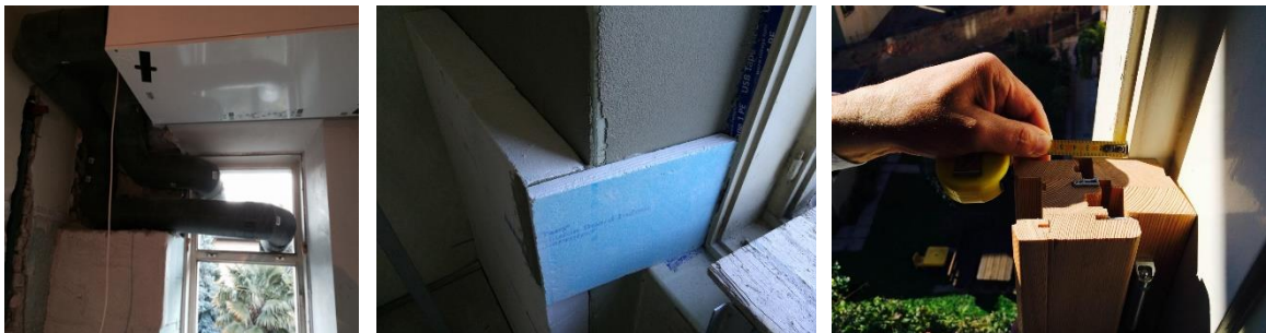
Figure 43: House Moroder, window details – before and after renovation.
