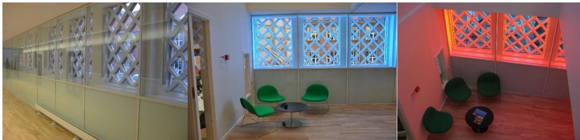
Figure 23: Left: Glazing layer added to inside of wall/window. Middle/Right: LED-lighting adds possibilities, © Wissenberg A/S
