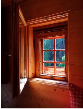
Figure 25: New opened window with the original window behind, ©Pavel Sevela
