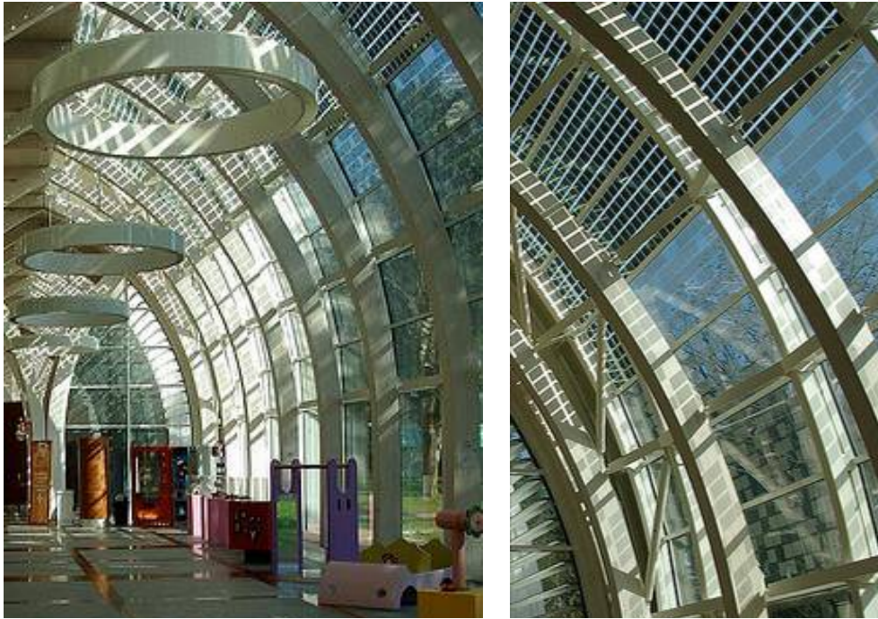
Fig. 3.B.22: semi-transparent skylights. Ospedale Meyer, Florence. CSPA Firenze, Paolo Felli, Lucia Ceccherini Nelli, Marco Sala: semi-transparent modules with crystalline cells. © Emanuele Noferini
