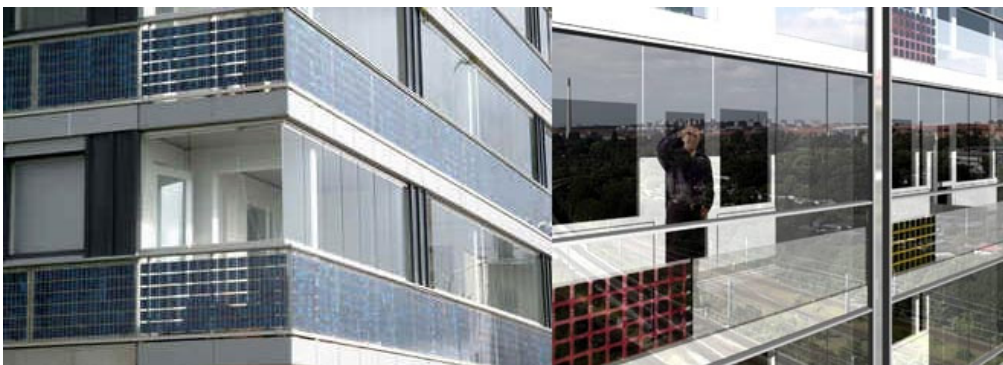
Fig. 3.B.30: spandrels and parapet solutions. Left: Housing Estate, Ekovikki, Finland, Oy Reijo Jallinoja: semi-transparent PV modules with two-paned glazing in parapet areas, Resource: PV NORD. Right: Kollektivhuset, Copenhagen, Denmark, Domus Arkitekter: PV cells were laminated to a single glass, heat transmitted from the cells was used in an innovative way to create thermal comfort during spring and autumn, during summer they are ventilated with an optimized shaft behind the cells and a coloured shutter through airgaps in the bottom and top of the glazing of the balcony, Resource: PV NORD.
