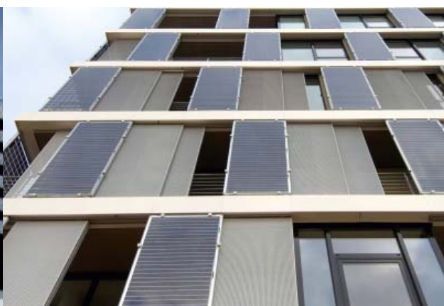
Colt Ellisse PV sliding shades at Company HQ, Bitterfeld-Wolfen, Germany, © Colt International Licensing Ltd., 2011
