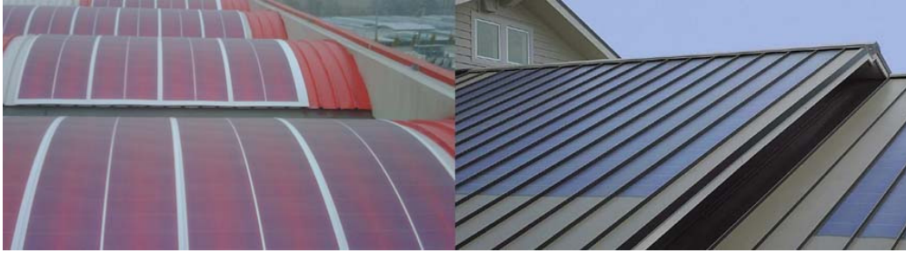
Fig. 3.B.39: flexible thin film laminates. Left: thin film laminate with plastic substrate using a galvanized steel plate to mount on a corrugated sheet curved roof, © Flexcell. Right: thin film laminate with stainless steel substrate glued on a standing seam metal roof, © Unisolar.
