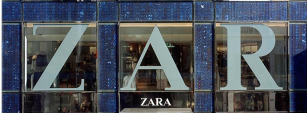
Fig. 3.B.24: warm façade solution. Zara Fashion Store, Cologne, Germany, Architekturbüro Angela und Georg Feinhals: opaque monocrystalline cells combined with transparent glazing in post-beam curtain wall structure, © Solon.
