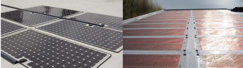
Fig. 3.B.20: integration of thin film laminates on flexible substrate in flat roof.
