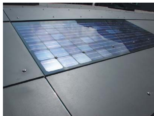
Photovoltaic INTEGRAL PLAN (SunTechnics Fabrisolar AG)
