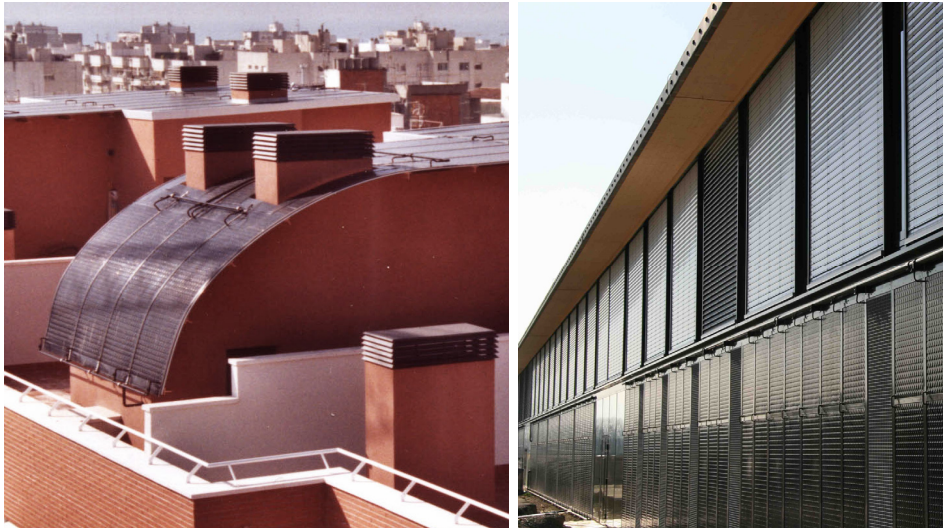
Fig. 3.A.15: Roof integration of unglazed flat plate collectors used as roof covering. Credits Energie Solaire SA
