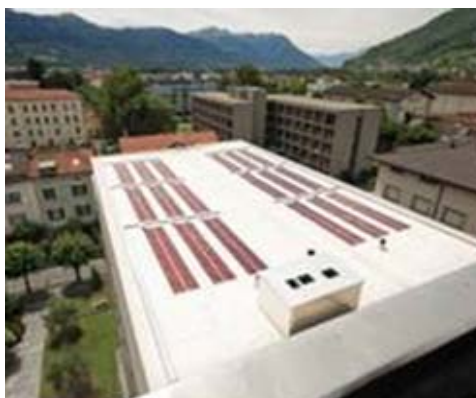
FLX-TO Installation - Bellinzona (CH), © VHF – Technologies
