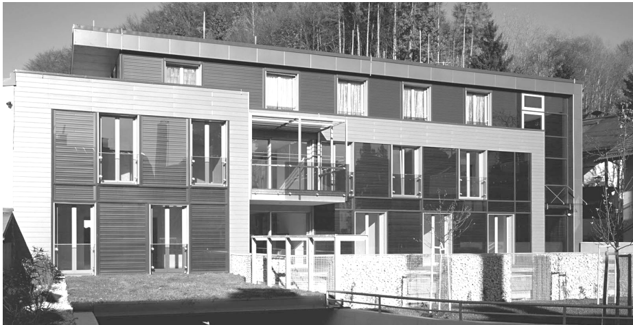
Fig. 3.A.11: Façade integrated solar thermal system. GAK Training centre in Graz, Austria. Arch: Josef Hohensinn
