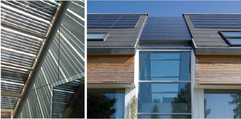
Fig.3.A.19: Evacuated tubes collectors used as glazed roof sunshading (left: inside view, right:outside view), Dubendorf Residential building, Beat Kaempfen 2008.
