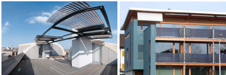
Fig.3.A.17: Evacuated tubes collectors used as deck sun shading. RaU Architekten. Credits: RaU Architekten.
