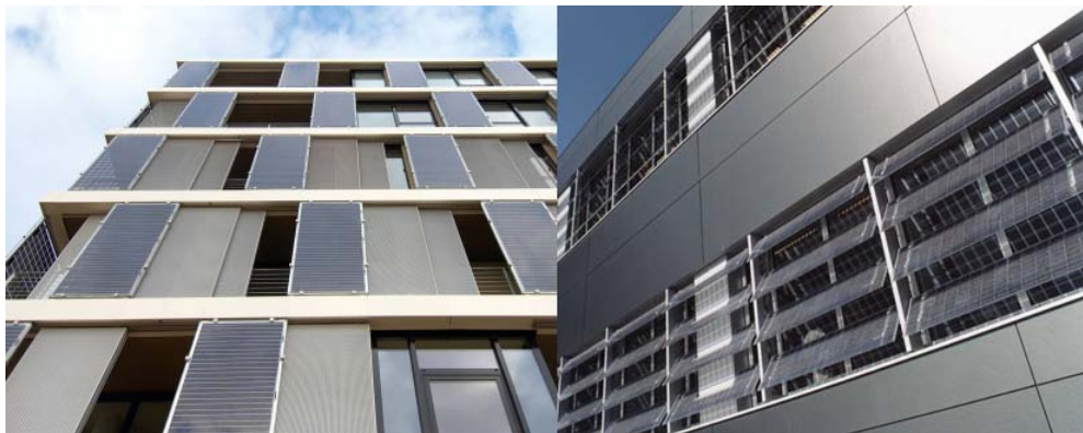
Fig. 3.B.28: solar shading solution: Left: Colt Ellisse PV sliding shades at Company HQ, Bitterfeld-Wolfen, Germany, © Colt, Right: Keuringsdienst, Eindhoven, The Netherlands, Yanovshchinsky Architekten: using Colt Shadovoltaic as shading device, © Colt.
