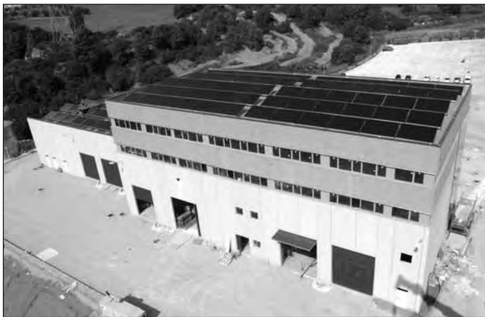
Figure 7. The Parking Service Castellbisbal SA facility for container washing in Barcelona, Spain. Source: Aguasol Engineering, Spain
