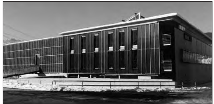
Figure 5. A solar heated production hall and office building in Doma, Austria
