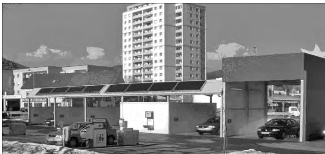
The Sunwash plant in Gratkorn, Austria
