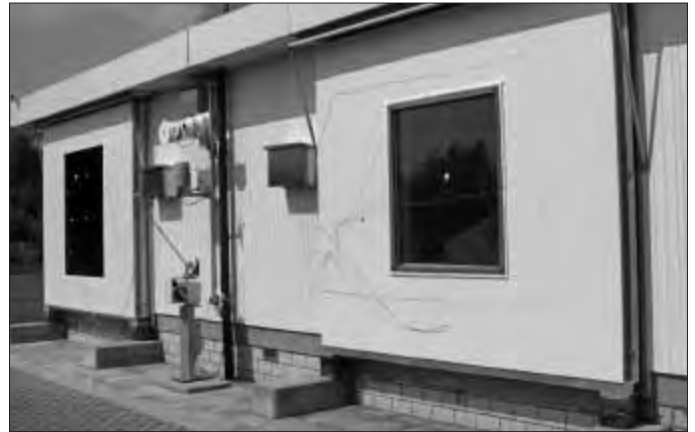
EMPA Test Cells in Duebendorf, Switzerland
