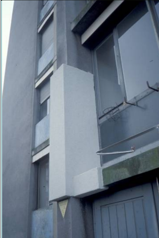
External insulation, test
