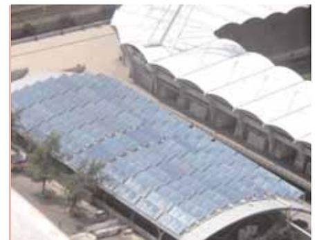
**Solar district heating plant in the city of Graz with an installed capacity of 1 MWth (1400 m<sup>2</sup> collector area).** (Source: S.O.L.I.D.)
