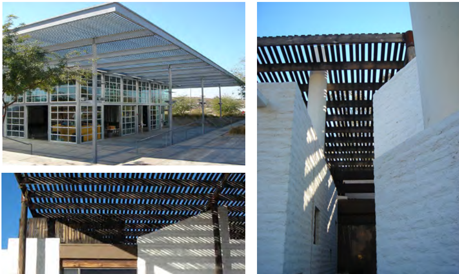
Fig. 3.A.20-a-b-c: Examples of double roofs conceived to reduce building heat (a: double tin roof in Arizona architect n.a; b and c: double roof on a private house in Arizona. Architect Judit Chafee, credits Marja Lundgren).
