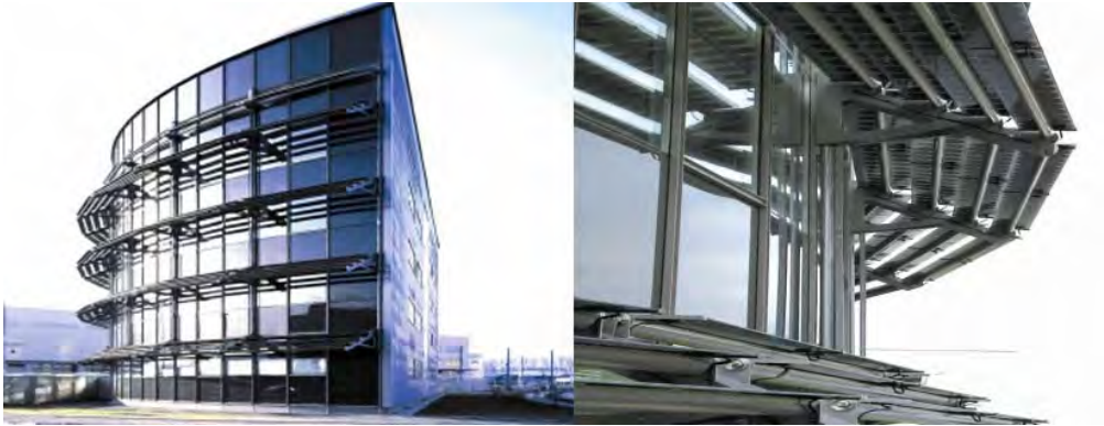
Fig. 3.B.29 SBL Offices Linz, Austria, Helmut Schimek, shading louvers with integrated photovoltaics and suntracking system, © Colt
