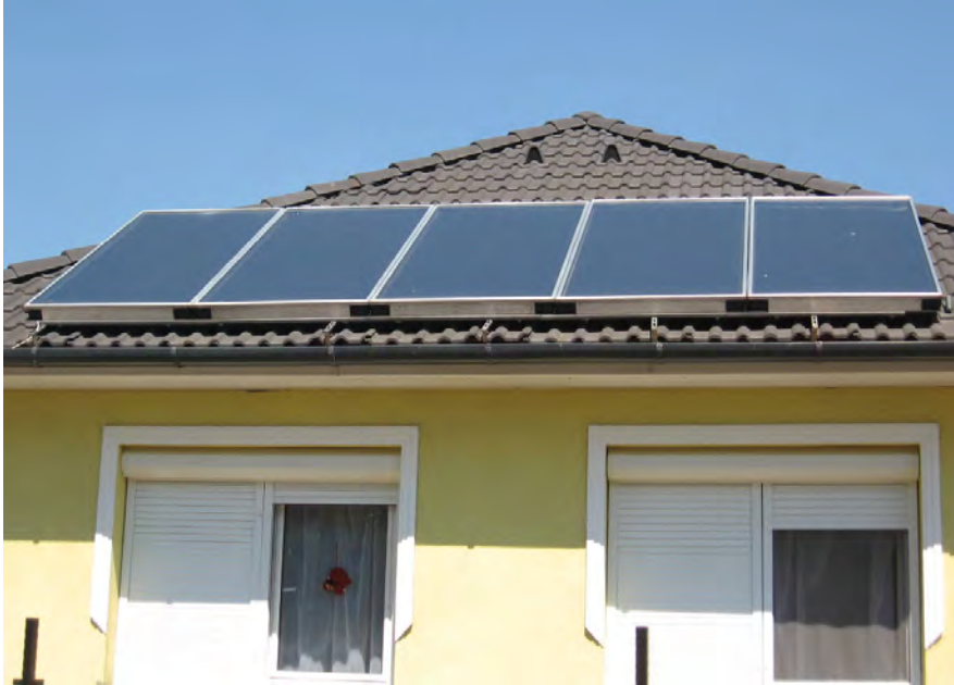
Fig. 3.A.21 Typical standard glazed flat plate collectors installed over the roofing, as purely technical add-on
