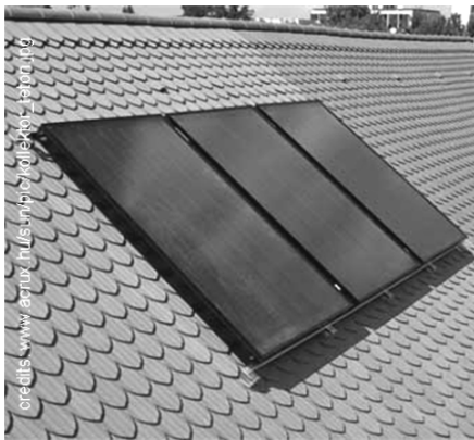
Fig 3.A.5 a- b: Glazed flat plate collectors applied on a tilted roof (left). Right: Typical glazed flat plate collector's cross section and main composition elements.
