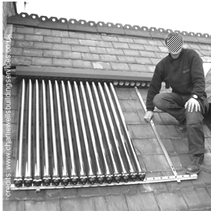
Fig 3.A.7 a- b: Vacuum tubes collectors mounted on a tilted roof (left). Right: typical vacuum tubes collector's cross section and main composition elements.
