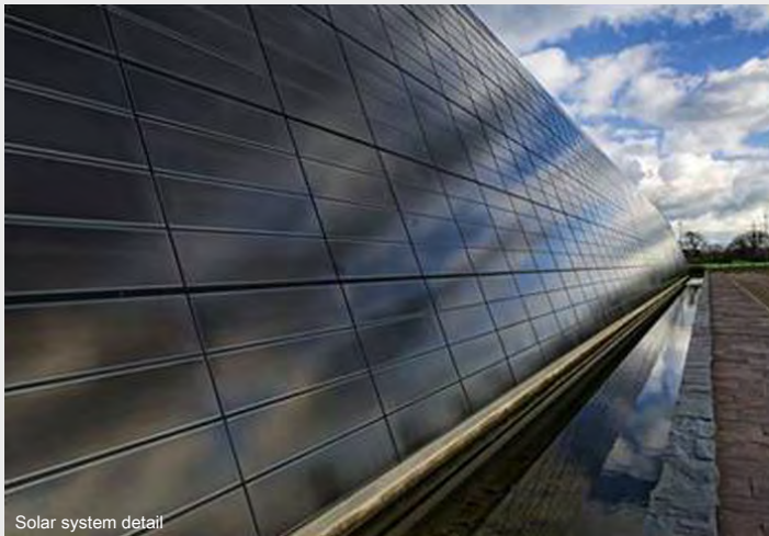
Solar system detail
