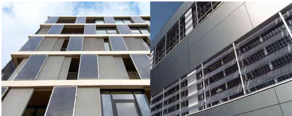
Fig. 3.B.28: solar shading solution: Left: Colt Ellisse PV sliding shades at Company HQ, Bitterfeld-Wolfen, Germany, © Colt, Right: Keuringsdienst, Eindhoven, The Netherlands, Yanovshchinsky Architekten: using Colt Shadovoltaic as shading device, © Colt.
