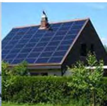
House in Cudrefin (FR-CH), © 3S
