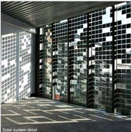
Solar system detail
