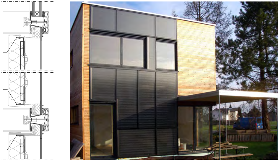
Fig. 3.A.14: Façade integration of glazed flat plate collectors as façade cladding, detail and picture. Credits AKS Doma, www.aksdoma.com
