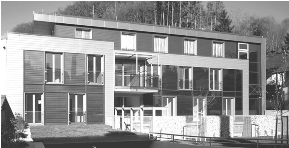
Fig. 3.A.11: Façade integrated solar thermal system. GAK Training centre in Graz, Austria. Arch: Josef Hohensinn
