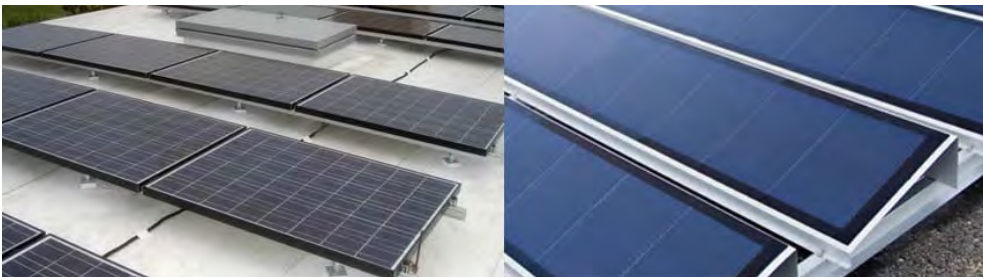
Fig.3.B.19: crystalline modules for flat roof. Left: standard module on rack mounting system, © Prosolar Right: special rack system for flexible laminate on stainless steel substrate, © Unisolar.
