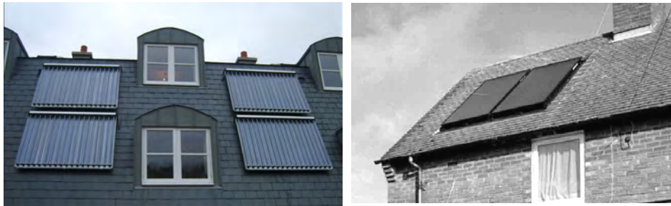
Fig. 3.A.12: Integration of collectors as added elements on the roof.
