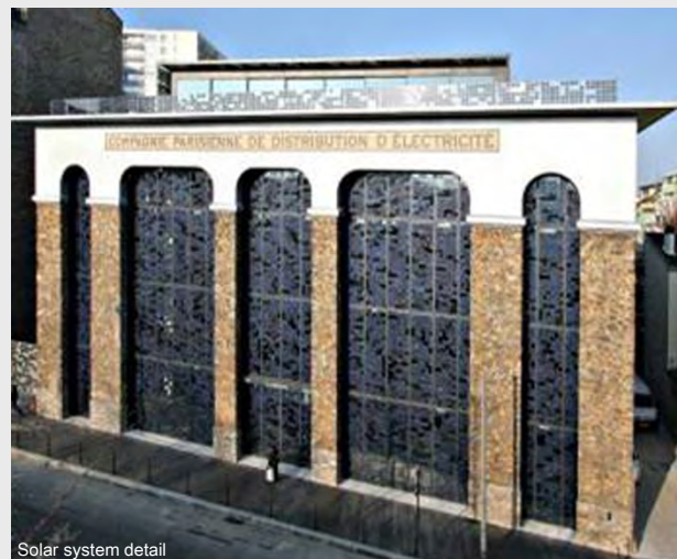
Solar system detail
