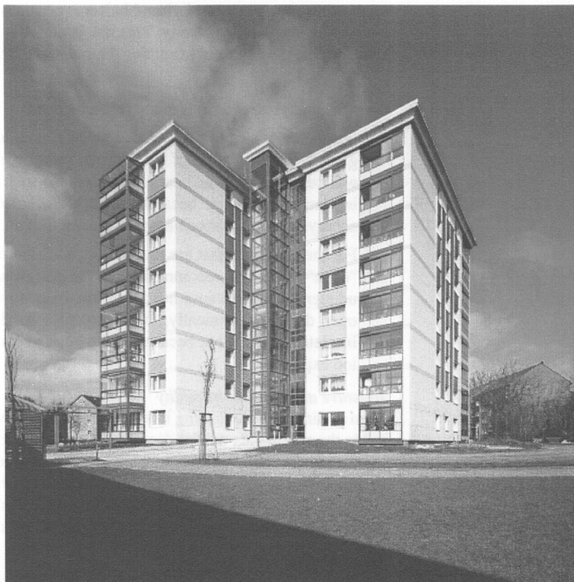
Figure 9: Picture of installed advanced glazed balconies, Engelsby – Flensburg.
