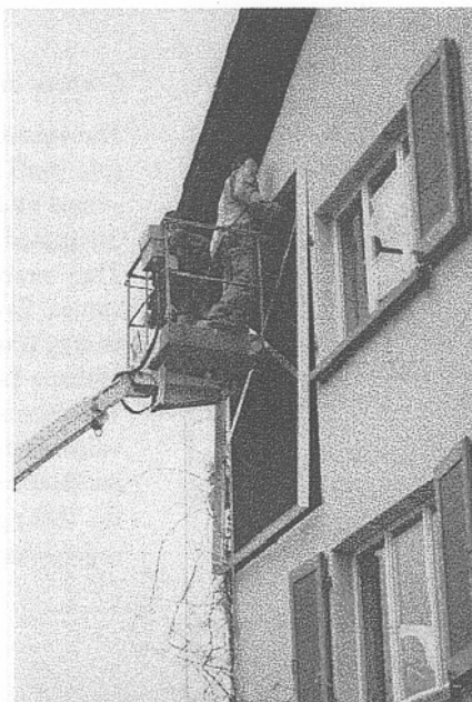
Figure 5: Installation of the prototype.
