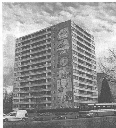
Apartment building in Freiburg, D, before renovation
