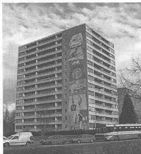
Figure 1: View of the apartment building Krozinger-Str. 4 before renovation.
