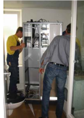
Installation of the combined heating and ventilation unit
