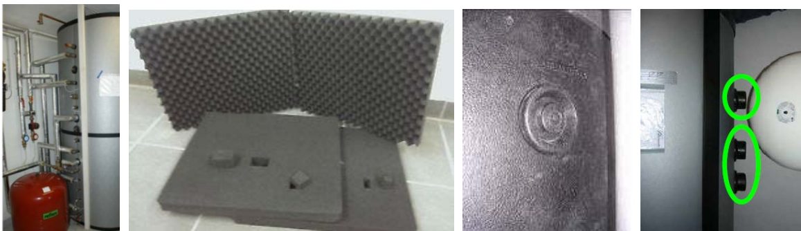
Fig 2. Tank pipe connections: bad example (left) and examples for improvements with pre-cut thermal insulation to be chosen when needed (middle) or insulation plugs for unused pipe connections (right) [4]
