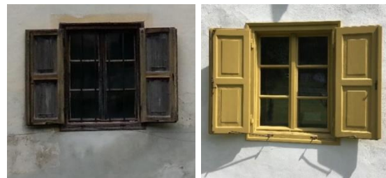
Knablhof (box-type window) – before and after renovation.
