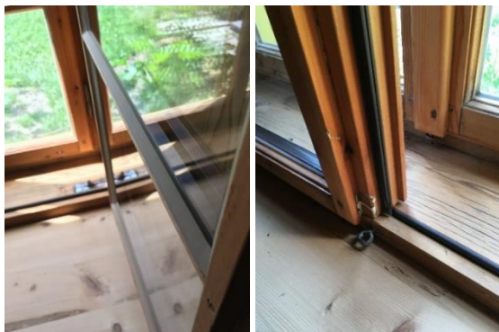
Knablhof (box-type window) – details after renovation
