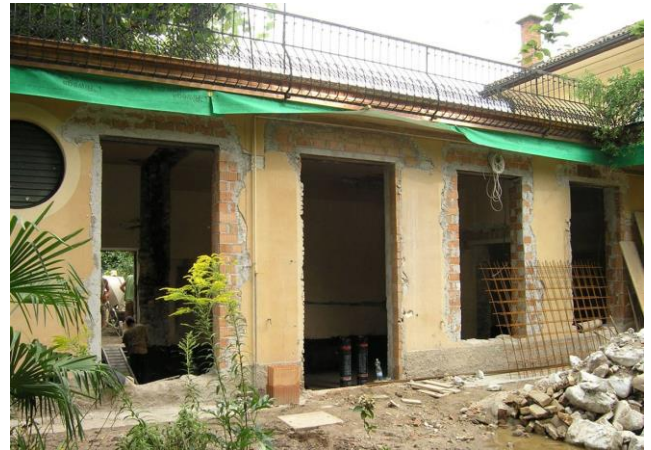
Ansitz Kofler during retrofit.
