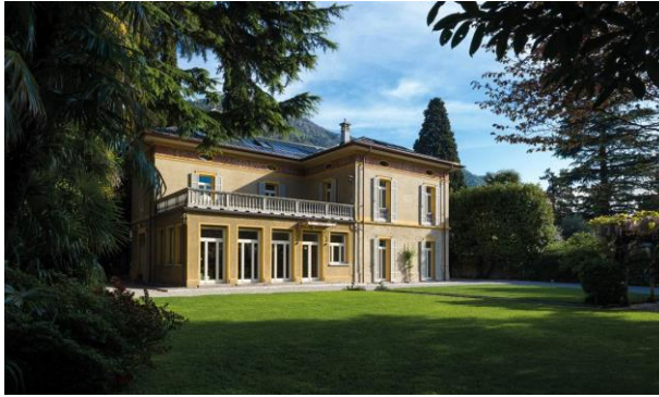
Villa Castelli, Bellani, Italy after the renovation that achieved a 90% energy demand reduction.
