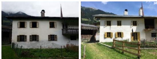
West view of Knablhof before and after retrofit
