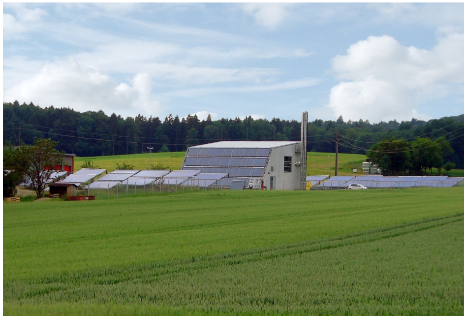
Fig. 9. Collector array and boiler house of Bioenergy Village Büsingen SDH (source: Solites).
