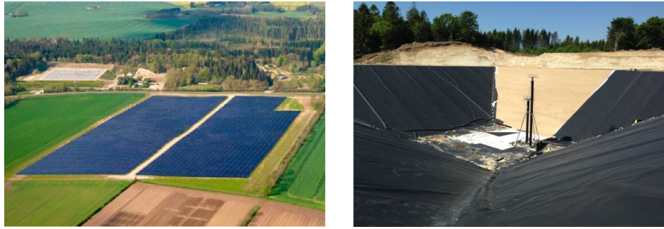
Fig. 3. Collector arrays (left) and PTES (right) of Dronninglund SDH (source: PlanEnergi).
