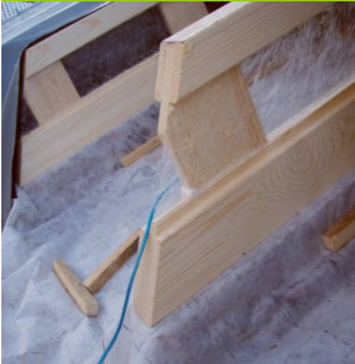
Roof Upsi framing
