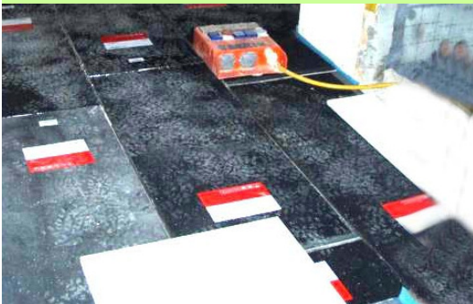
Vacuum insulation panels VIP on floor
