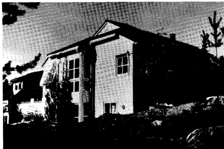
4.4: Passive Solar Home, Oslo, Norway
