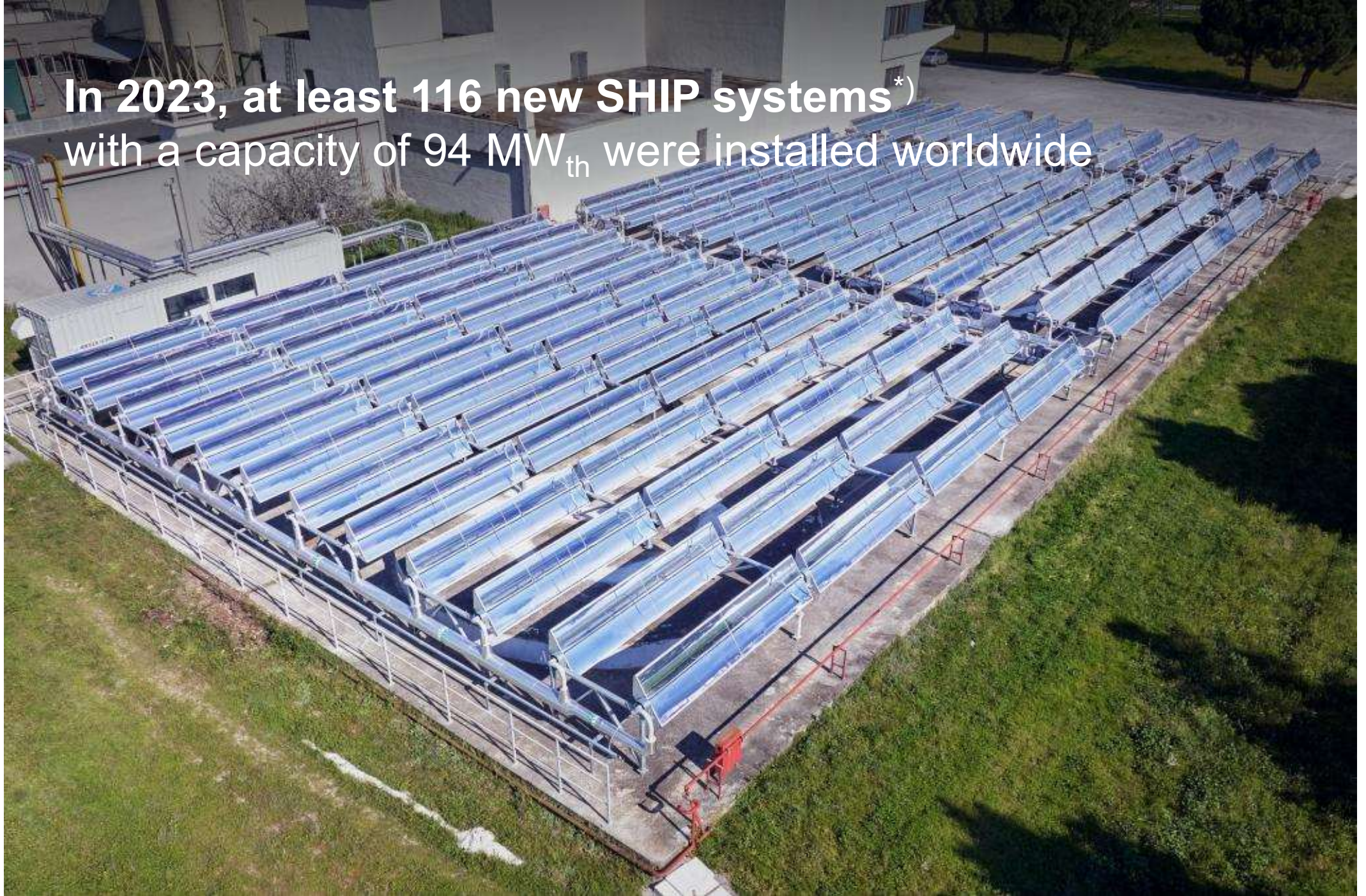
Parabolic trough collectors for one of the breweries of the Carlsberg Group in Salonika, Greece
