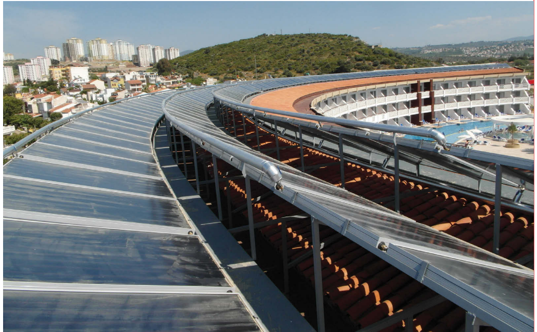
▲ Solar thermal application for hot water production at the Ephesia Hotel in Kusadasi on the Aegean coast.
