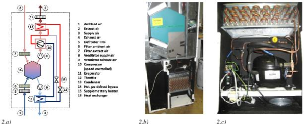
Figure 5. a) Hydraulic scheme of the micro-heat pump; b) photo of MHVR (Pichler Luft) and evaporator (Siko Energiesysteme) c), compressor and condenser (Siko Energiesysteme).
