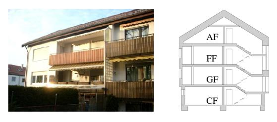
6.a) 6.b) Figure 11 a) South façade of the existing multi-family house, with adjacent neighbouring building, b) section after the renovation; CF: cellar floor, GF: ground floor, FF: first floor, AF: attic floor, Wohnungsbau Ludwigsburg
