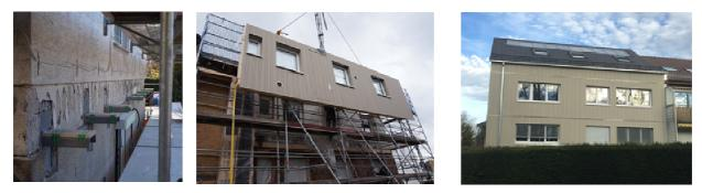
Figure 8.a) Steel supports of the timber frame wall
