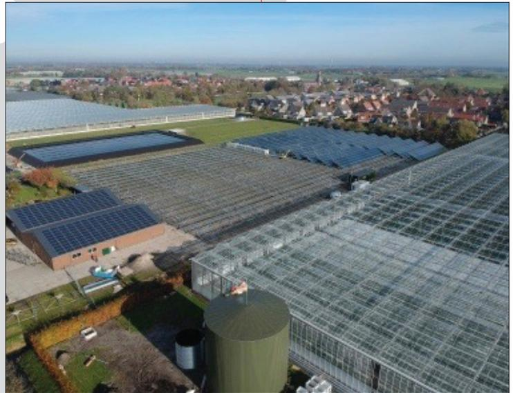
▲ **The largest solar thermal system in the Netherlands is for heating the Tesselaar Freesia Heerhugowaard greenhouse. The system has 9,300 m<sup>2</sup> of collectors with two storages, a 30 m<sup>3</sup> basement return vessel and a 1,400 m<sup>3</sup> storage tank. The overproduction of heat during summer is stored in the soil.** (Source: G2 Energy)
