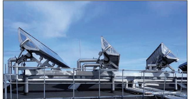
▲ **Concentrating solar collectors supply heat and steam to power absorption chillers for the Härnösand hospital's radiology department in Sweden.** (Photo: Absolicon)
