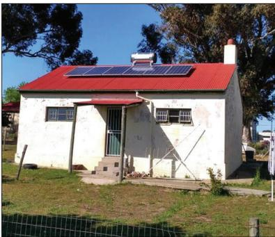
▲ **PV2heat system at the Mariendal Experimental Farm of Stellenbosch University in South Africa consisting of 1.5 kW<sub>peak</sub> PV and a 200-liter hot water tank.** (Photo: SOLTRAIN)
