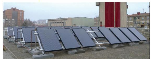
▲ **Figure 4.** In Spain, 28 PVT glazed panels covering 46 m<sup>2</sup> generates 6.7 kWp for DHW in a firehouse. Electricity is for self-consumption and the grid. (Credit: Endef Engineering)
