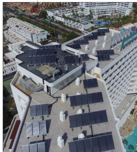
◀ In Spain, the conditions are suitable for a low payback time. 102 PVT glazed panels covering 200 m<sup>2</sup> generate 30 kWp to provide hot water and electricity for self-consumption and the grid at this hotel. (Credit: Abora Solar)
