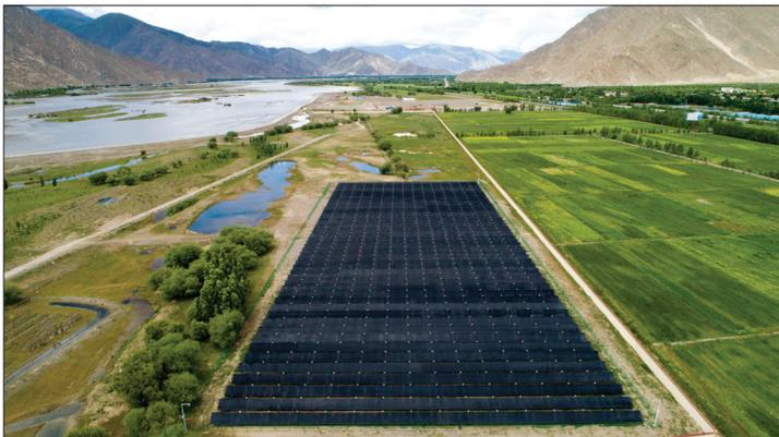
▲ **Lasha solar district heating system in Tibet, China, with 11,250 m<sup>2</sup> collector area (9.1 MWth).** (Photo: Solareast Holding Company Ltd.)
