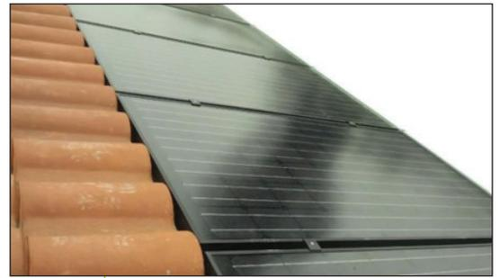
▲ **Figure 2.** In France, six PVT uncovered panels, 9.6 m<sup>2</sup> and 1.5 kWp, for domestic hot water preparation, heat for a heat pump, and electricity for self-consumption and the grid. (Credit: Dualsun)
