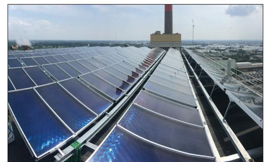
▲ **Large-scale flat plate collectors for an industrial application feed into the district heating network in Vienna, Austria. The 656 m<sup>2</sup> collector area, located on a 70 m high roof of an existing boiler house, produces 780 kWh/m<sup>2</sup> annually.**
