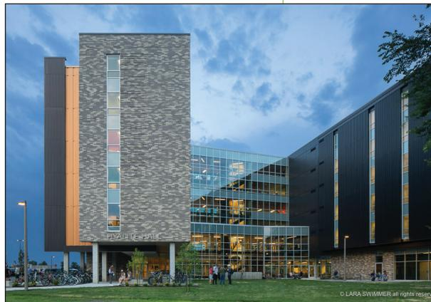
◀ **0.6 MWth façade integrated solar air system at Montana State University in Bozeman, Montana, USA.** (Photo: SolarWall)
