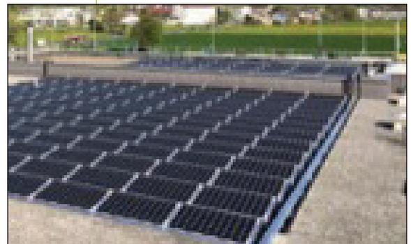
▲ **Figure 3.** In Switzerland, this PVT system uses 178 uncovered PVT panels + 699 PV modules to generate 237 kWp. The heat pre-heats the groundwater storage, which is then transferred directly to the heat pump and the overflow basins of the pools. The heat pump generates heat for pools, space heating, and domestic hot water. A gas boiler supports the heat pump for peak loads. Electricity is for self-consumption and the grid. (Credit: Meyer Burger)
