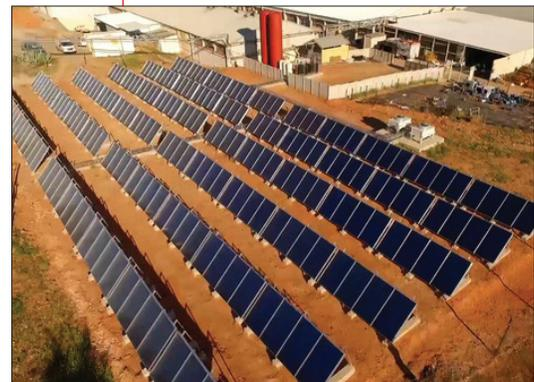
▲ **Klein Karoo International (Pty) Ltd Tannery (KKI) installed a solar thermal plant. In one year, this solar installation generates 397 MWh and is responsible for avoiding 137,000 kilograms of CO<sub>2</sub> emissions.** Source: SOLTRAIN
