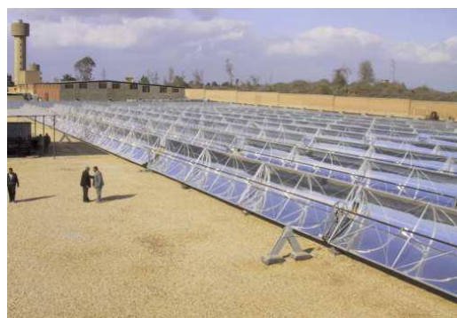
Fig. 12: Solar thermal process plant - steam production in chemical industry (source: Fichtner Solar GmbH, Germany)
