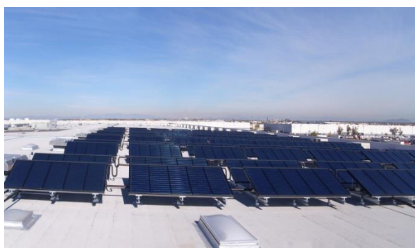
Fig. 13: Solar thermal process plant- hot water production used in the beverage industry (source: SOLID GmbH, Austria)
