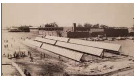
First solar thermal district heating plant at Northview Junior High School (USA) designed and installed by Honeywell in 1974.
