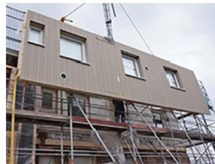
The objective of the EC-funded project iNSPiRe is to reduce the problem of high-energy consumption of existing buildings by producing systemic renovation packages that can be applied to residential and tertiary buildings. The renovation packages aim to reduce the primary energy consumption of a building to lower than 50 kWh/(m<sup>2</sup> a) for ventilation, heating/cooling, domestic hot water and lighting.
