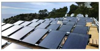
A PVT field of collectors on a flat roof is not different from a T field or a PV array. Integrated solutions will look totally similar to PV-only solutions. *Credit: Endef - Spain*
