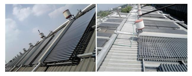
Figure 9: Evacuated tube collectors on the roof of Wheels India in Padi, Chennai, with a collector gross area of 1,365m<sup>2</sup> (Source: IEA SHC Task49 & SoPro India)
