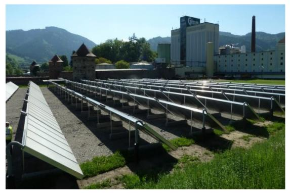
Figure 6: Flat-plate collector field with 1,500 m<sup>2</sup> at the Goess Brewery (Source: AEE INTEC)
