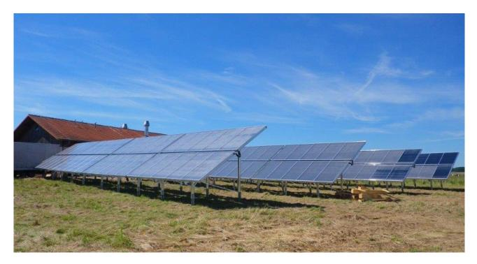
Figure 1: Field of flat plate collectors close to the GPRS building (Source: Enersolve)
