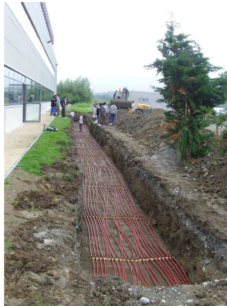
Fig. 12: Example of horizontal ground probe heat rejection system in INES office, Chambéry (source: INES RDI)
