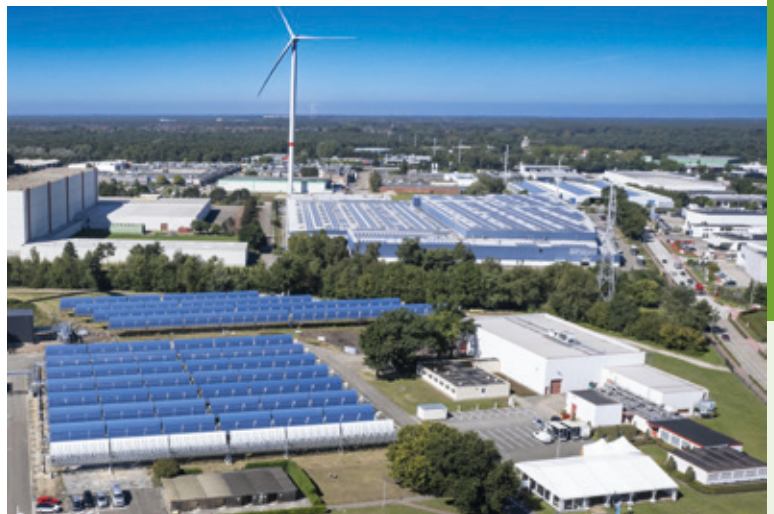
3.9 MW th Parabolic trough collector system at the company Avery Dennison in Turnhout, Belgium
