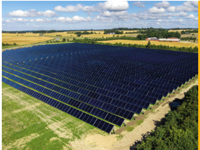
Solar district heating Jelling, Denmark Photo: SavoSolar / Solar Heat Europe
