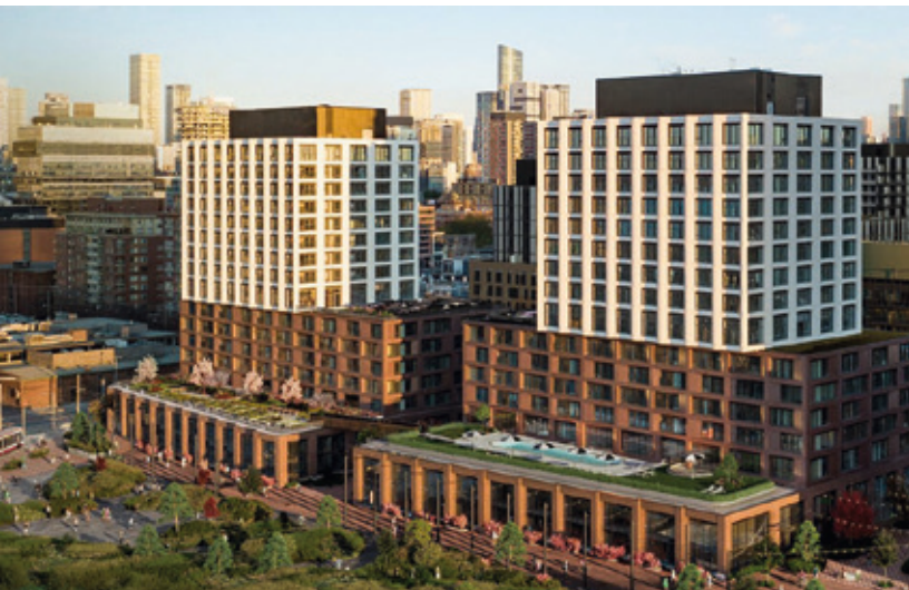
Solar air heating systems on the mechanical room penthouses at the Canary Commons, a condo community in Toronto, Canada Photo: SolarWall Conserval Engineering Inc.
