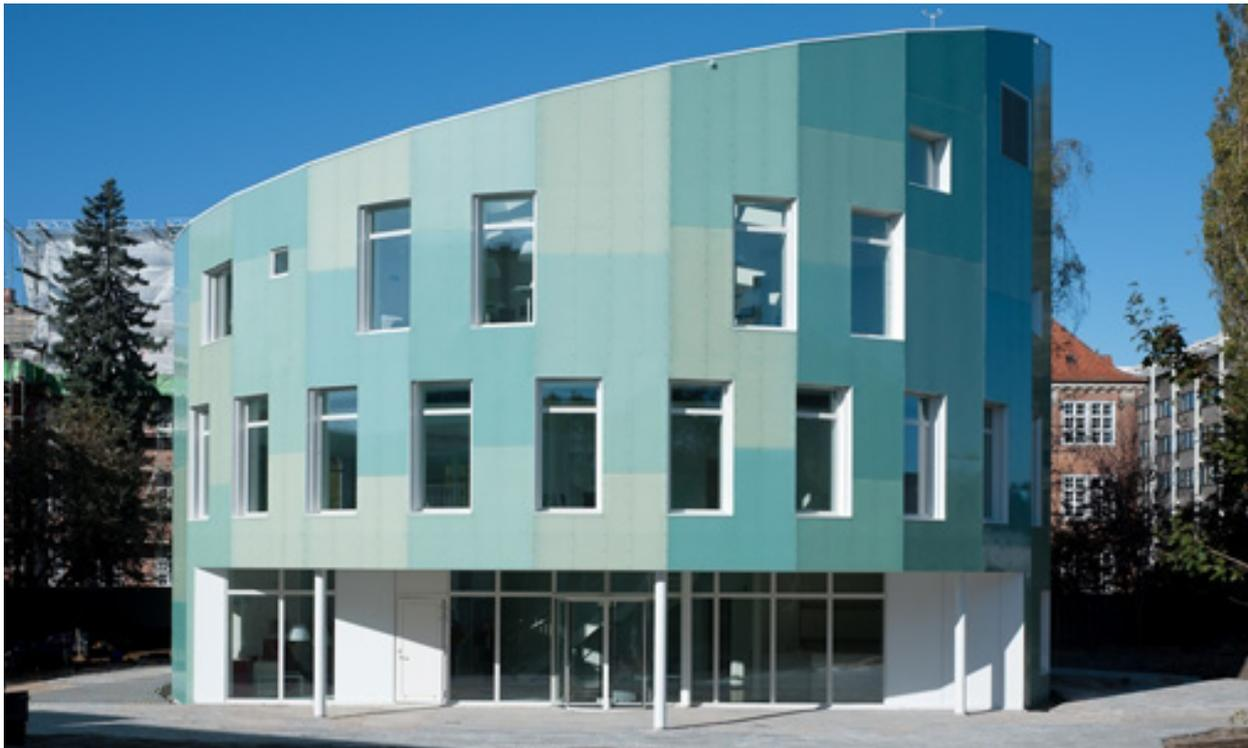
ambitious goal of reaching a low-energy building on the levels of the 2020 building regulations. The project team focused mainly on using the sun as a primary energy source to heat and light the building, including a strategy for well-insulated walls, solar shading, and solar panels to provide electricity. A circular shape was chosen in order to save material and to be able to fully exploit the course of the sun in the context of the building.
