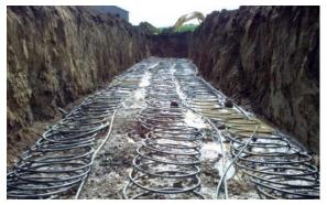
Figure 18: Geothermal Heat Pump - Horizontal Trenches<sup>36</sup>
