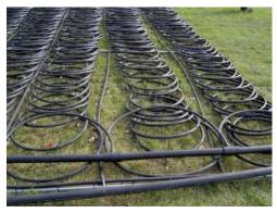
Figure 17: Closed System<sup>35</sup>
