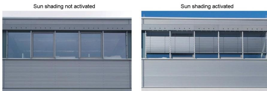
**Figure 17:** Photographs of the façade operating modes considered in a façade status-related, relative usable luminous exposure
