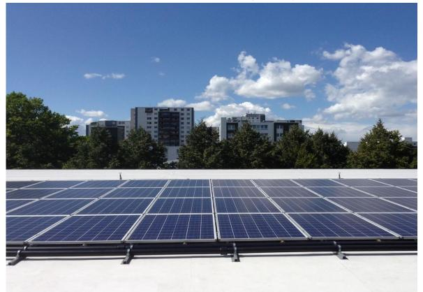
Double use of the surface to produce electricity and heat.
